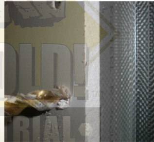
Drill 1/2" hole through stud
