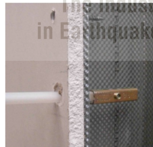
Push Toggler through hole
