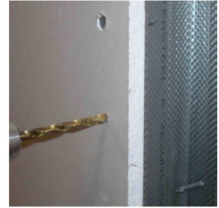
Drill 1/4" hole ending when stud is hit
